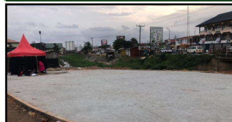
Effia Events Grounds Pavement Project ( Ongoing )
