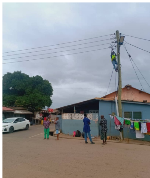
Street lighting project
