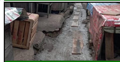
Concreting Effia Market Walk Ways
